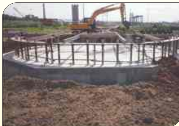
Civil & Strl. Works for U&O (M/s CINDA): Flare stack foundation
